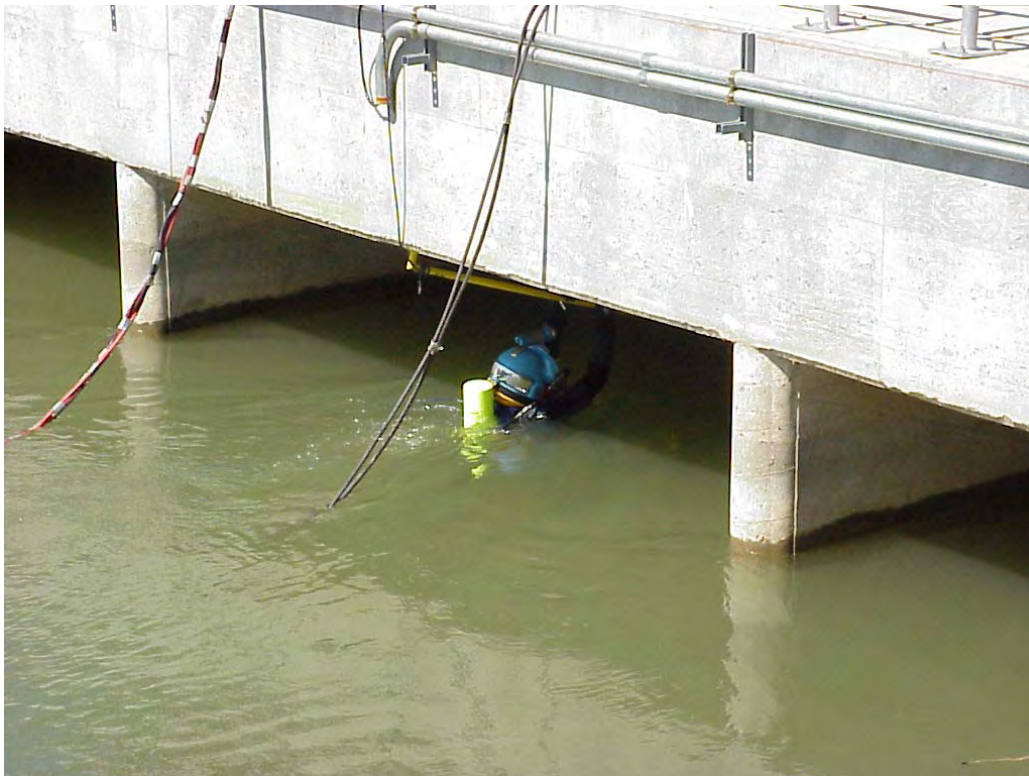
Figure 4. Diver descending into channel using the installed handrail.
