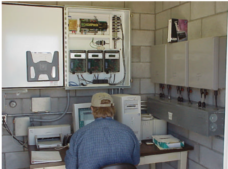
Figure 3. Housing structure at GCID Stoney Creek Siphons site
