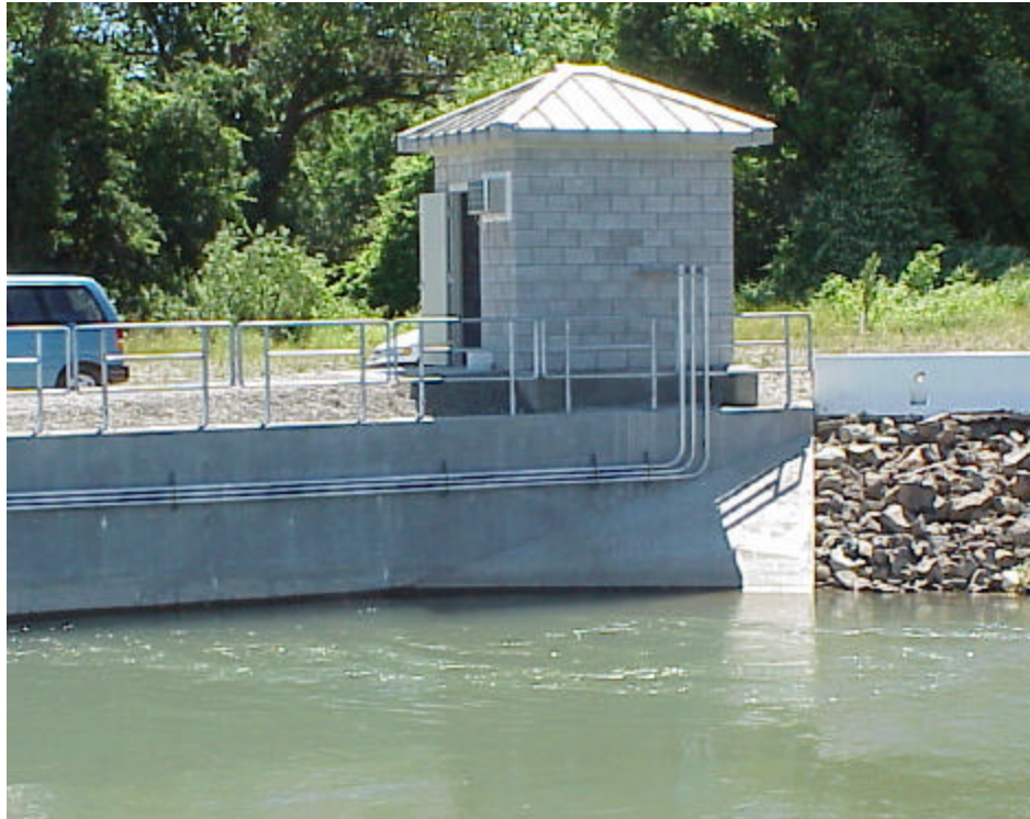
Figure 2. New flow-measurement structure at GCID Stoney Creek Siphons site
